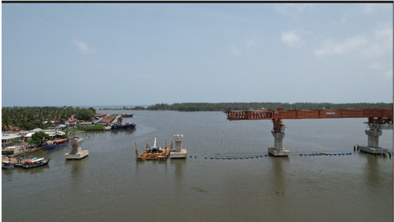
Azhikhode Munambam bridge work in progress
